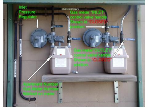
Gas meter control valve in closed position: When handle is across pipe it is CLOSED.
